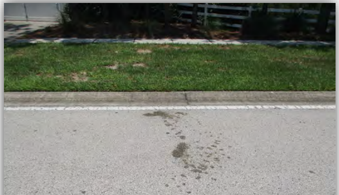
Adjacent to the SHBlvd. lift station approaching the south intersection from the north. Turf damage + hydraulic fluid leak.
